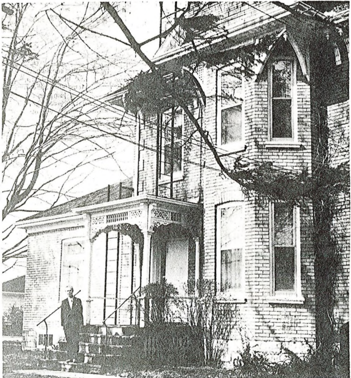
The building in use for Faith Haven was once a nursing home, and contains safety features such as emergency lighting and smoke detection systems, ideal for a resident school.
